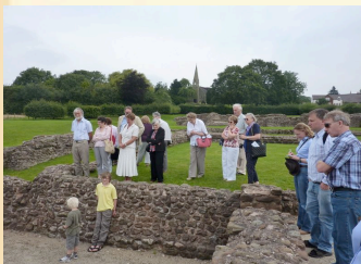
WHG members and friends inspect the footings at Wall
